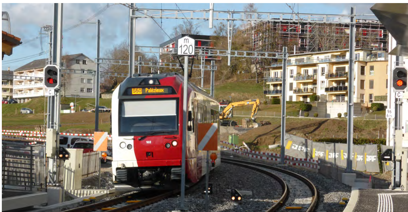
Châtel-St-Denis station on 6 March 2020. Some construction was still under way. All photos Daniel Pixley except as noted.
